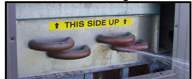
Freeze Damage
